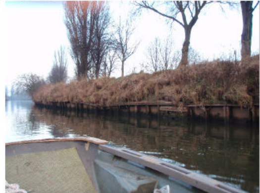
Downstream length: general view
